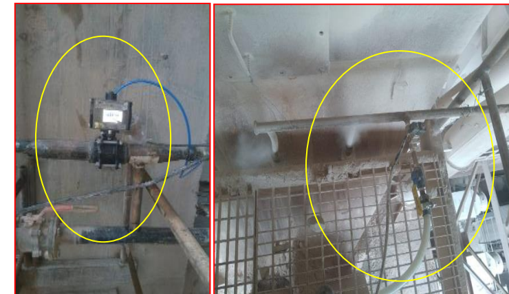
Water spray system provided for both raw mills.
