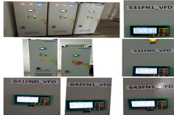
VFD INTALLED FOR 5nOS BAG FILTER FANS AT CM & PP
