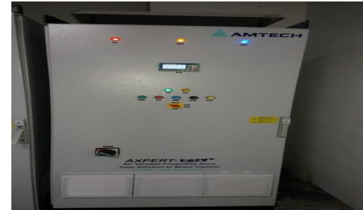
VFD INTALLED FOR CEP PUMP AT WHRPP
