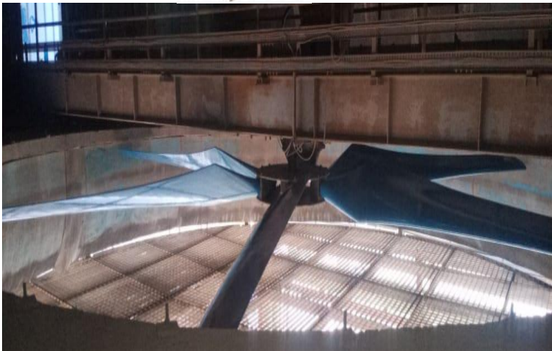
Replacement FRP Blades in ACC Fans- CPP (5062 kW/day saving, Invest 16.5 L)
