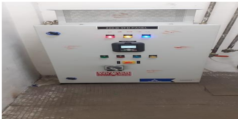
VFD INTALLED FOR RO WATER PUMP AT WTP
