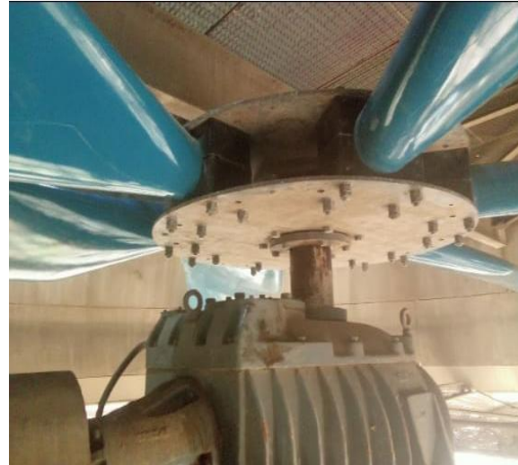
Replacement FRP Blades in ACC Fans- WHRP (1745 kW/day saving, Invest 12 L)
