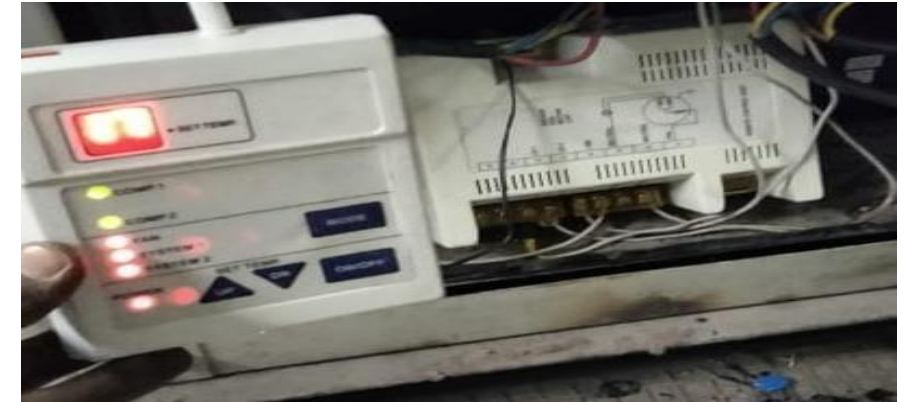
Universal Controller Kit for Package AC units at various location in plant area
